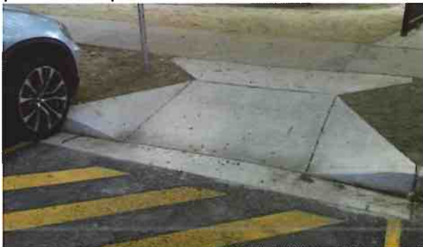
Suburban Kerb Ramp – Hall Street, Turner
